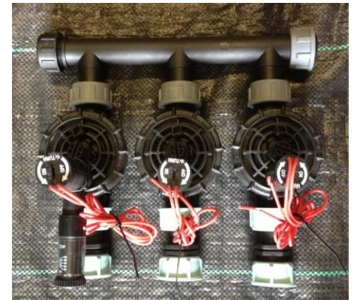
**After finally checking all fittings for security cover the solenoid manifold with the chamber, ensuring the valves will still be accessible from the inside. Fold the root guard matting upwards and use to seal the chamber orifices, then backfill around the chamber pressing the soil firmly and securing the chamber. (ensure the box lid is level with surrounding areas).**
