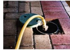
guaranteed regardless of the demands on the mains water system. Watering is also speeded up as the take-off points can be located at regular intervals around the areas to be watered, minimising the use of long hoses.
