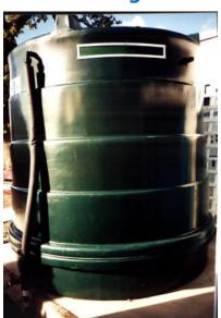
Water storage tanks are needed primarily to provide a 'type A' air gap in line with Water regulations. For many irrigation projects, the system can be designed to use water more slowly than it enters the tank from the public mains. In this case the tank only needs to be small.
