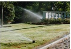
from within the lawn when watering commences. Inside each sprinkler there is a gear drive which causes the sprinkler head to rotate back and forth.
