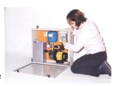
Modern electric pumps are compact and very reliable, smaller pumps are normally aligned horizontally, with larger pumps installed vertically. The pump is turned on and off by the control panel. An emergency stop switch would be located adjacent to the pump to comply with IEE regulations.
