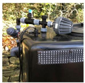
Designed for situations where on-site pressure is too low, or where Water Regulations demand Category 5 water protection. Pre-assembled pressurisation unit enabling easy installation and minimum on site work. The unit is pre-wired and tested at manufacture ensuring on site commissioning time is greatly reduced.
