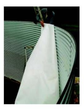
4. Work around the tank overlapping on the vertical seam by 25cm until the steelwork is completely covered by the fleece.
