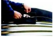
6. When the liner is free of creases, fit the outer split capping, removing the temporary clips as you go. The outside flap should be even all round; if it is not the tank is oval.
