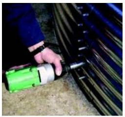
Check again for ovality; when all panels are in place tighten all the nuts and bolts. Fix the anchor brackets to the concrete base.
