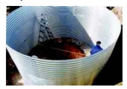
7. Second, third and fourth steel rings: Each additional ring of panels is fitted outside the ring below, thus creating an external overlap, enabling rain to be shed.
