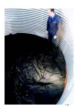
3. The person inside the tank passes up the edge of the liner to the outside man on the ladder who pulls the liner up until he has approximately 300mm of liner hanging down the outside of the tank, which he should secure with 75mm pieces of outer capping.
