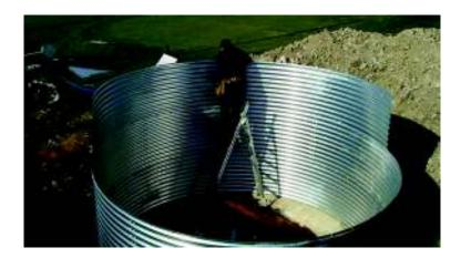
It is essential that each alternate ring is staggered i.e. the end of each panel should rest towards the middle of the panels below, similar to a brickwork effect.
