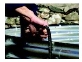
2. Roll out the liner over the 50mm sand base, laying it out so that the base to wall circumference seam is touching the steelwork all around. The vertical side will then be laying flat on the base. BEFORE working with the liner check the sand for stones or sharp objects. Also check your SHOES.
