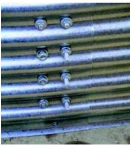
5. Fix the anchor brackets provided on the outside of the tank at each vertical end joint in the base ring, using the long bolts (M10 x 40mm) and additional spacer nuts. Do not fix the brackets to the concrete.
