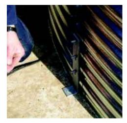
6. Check for ovality and adjust accordingly to provide a circle of the correct diameter. Tighten some of the bolts to hold the panels securely. Do not tighten all the nuts and bolts until the tank is fully erected.
